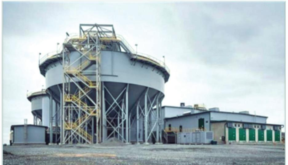
Thickener paste for optimal water recovery from tailings
